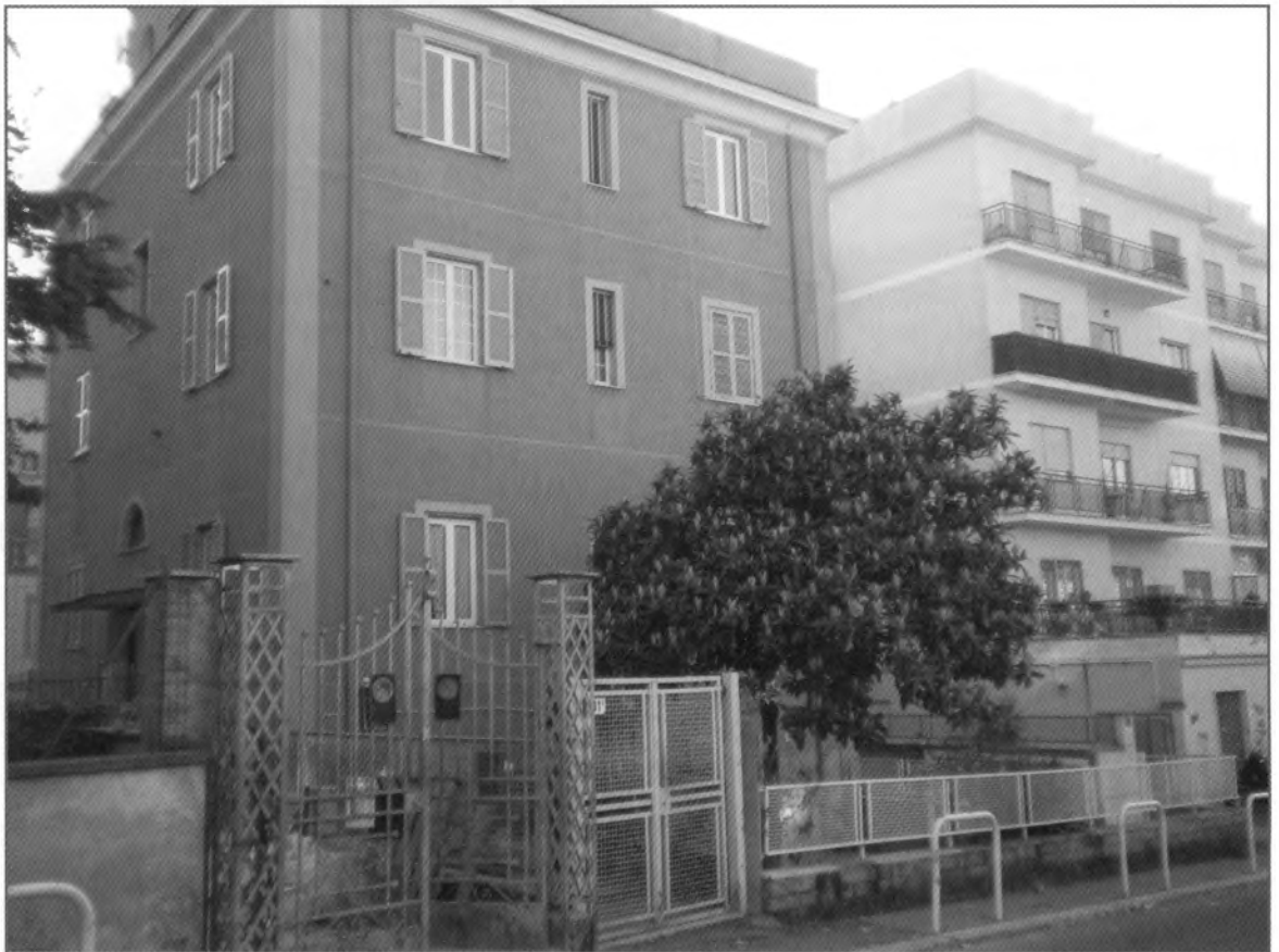
The apartment is located on the ground floor of this building
